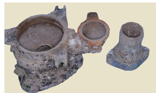
with galvanic anode installed
